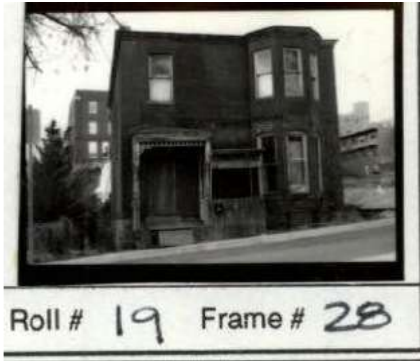
This ca. 1989 photo from the Historic Inventory Form shows what is very likely the historic porch. Note that the sheet metal in place over the brick between the second story single southwest window and the bay.
