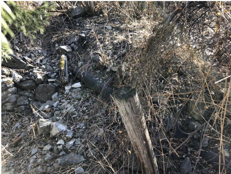
Figure 7 – Existing Above Ground Ductile Iron Pipe
