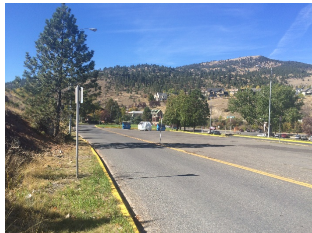
Cruse Avenue to form on/off ramps Note: Use of empty space for recycling containers
