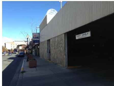
Parking lot structure on Last Chance in retail core of historic Downtown
