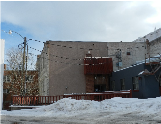
View from Fuller Avenue of a double-frontage lot with store front on North Last Chance
