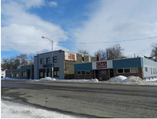
Helena Avenue near five-point intersection
