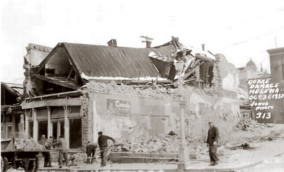
1935 Earthquake damage (Source: helenahistory.org)
