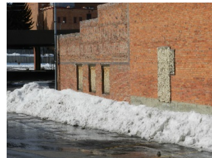
Located within historic downtown core
