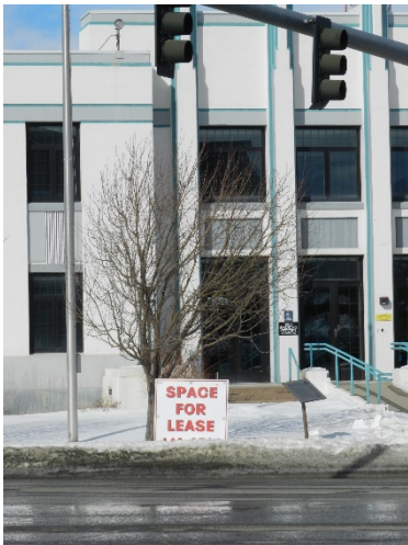
Armory Building at Lyndale and Last Chance
