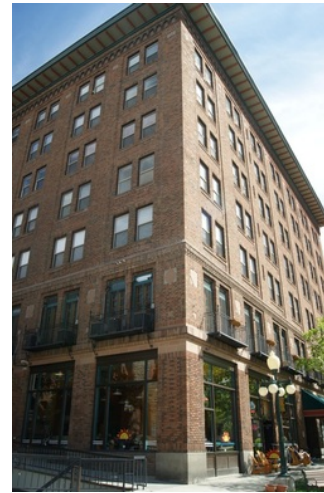
Example of a cornice at the top of the building (Placer Hotel)
