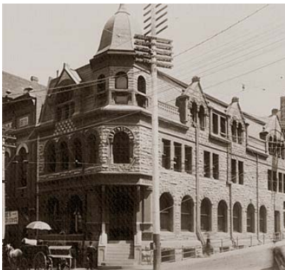
Original Securities Building, built with local stone and red sandstone from Bayfield, WI (Source: helenahistory.org)
