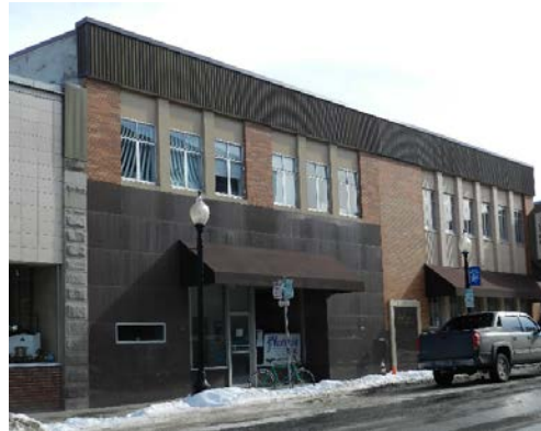
Building on Last Chance with various types of cladding
