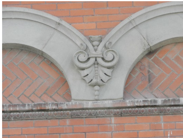
Example of architectural detail exposed when cladding removed (Fuller Street)
