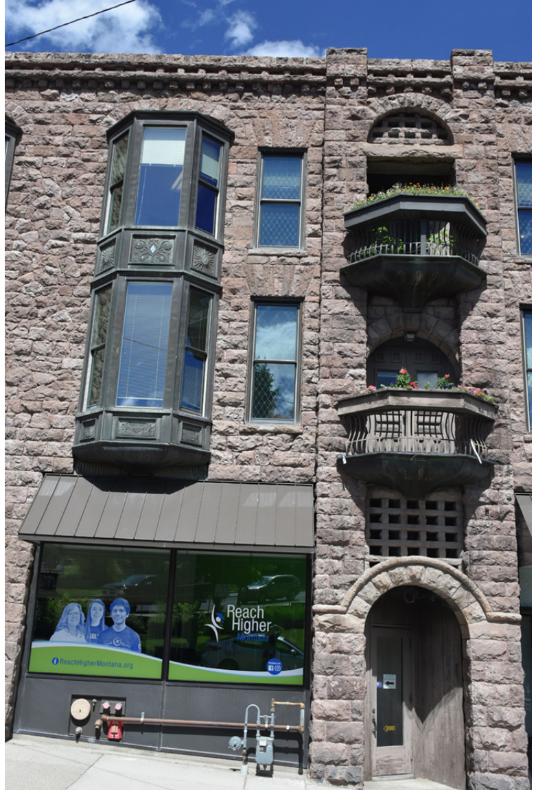
Figure 4.03 – Downtown and elsewhere, mixed-use buildings are seen as an effective strategy for Helena's housing objectives. (Image: SCJ Alliance, Inc.)
