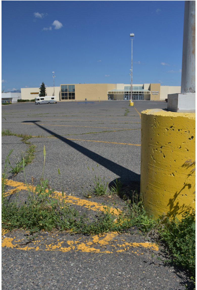
Figure 3.03 – Economic and land-use objectives in this plan support infill and revitalization efforts, creating growth while minimizing the community's physical "footprint." (Image: SCJ Alliance, Inc.)
