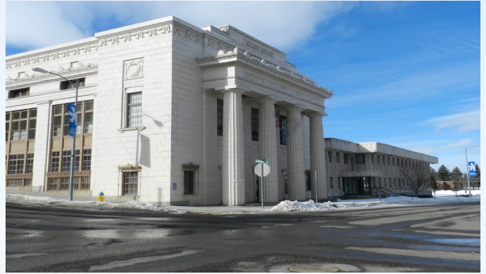
Vacant or underutilized buildings contribute to blight conditions in the downtown area.
