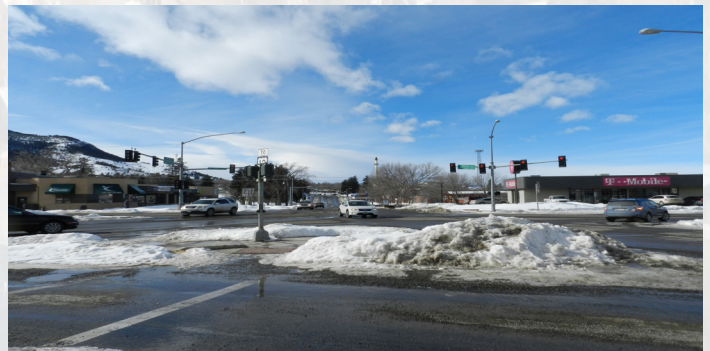
Five point intersection at Cruse, N. Last Chance, Neill and Helena Ave. creates congestion and circulation issues in downtown
