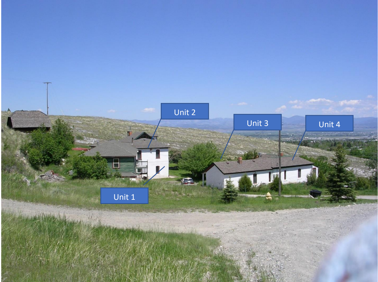
View of 304 Clancy from the south.
