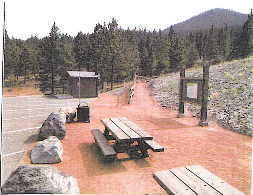
Beatie Street Trailhead Crushed Rock Fines that were installed by a City of Helena contractor to provide accessibility to trailhead amenities
