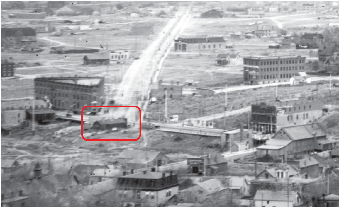
The rear 1/3 of the building was clearly built later as the roof structure is a more modern steel "bow" truss. In this image of the laying of the cornerstone of the Civic Center from 1920 the Livery building clearly was in existence prior to the rear addition.
